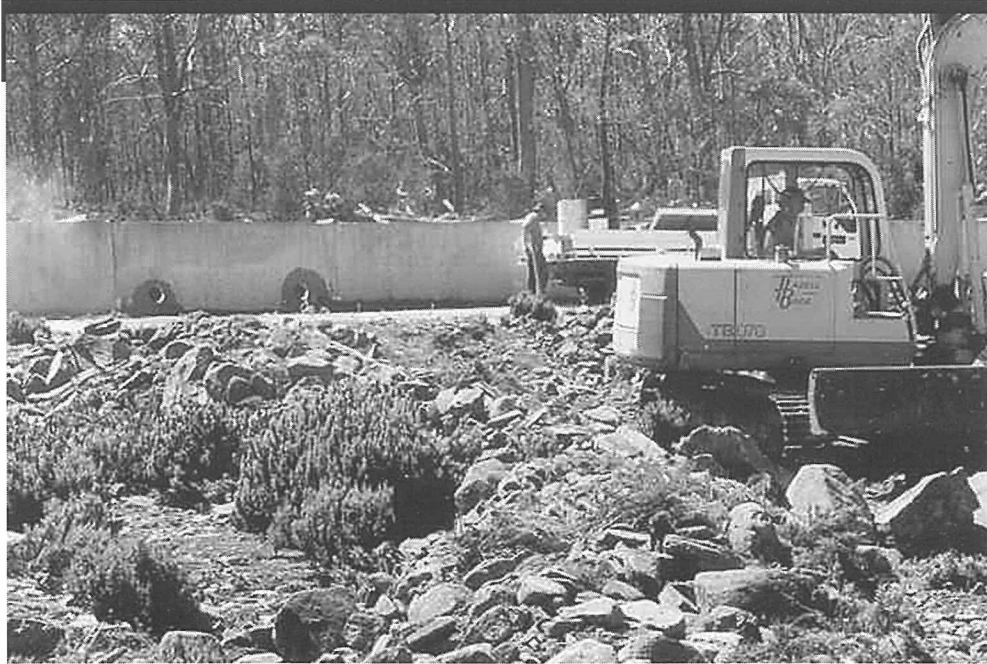
Flume excavations, allowing the release of water into the Ripple Creek catchment
