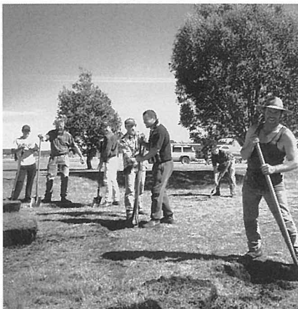
Longford Club members starting the building of the machinery shed, Liawenee
