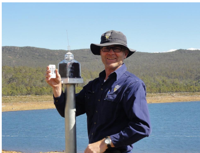
IFS Manager of Anglers Access, Neil Morrow, changing navigation light batteries
