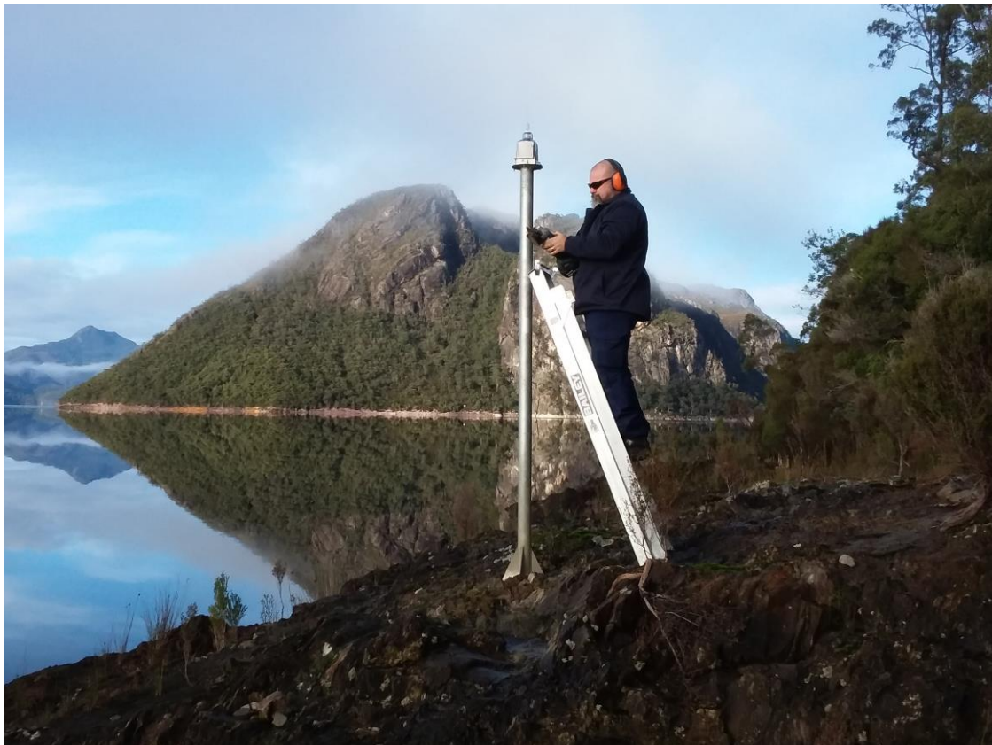
Installing a navigation light at Lake Mackintosh
