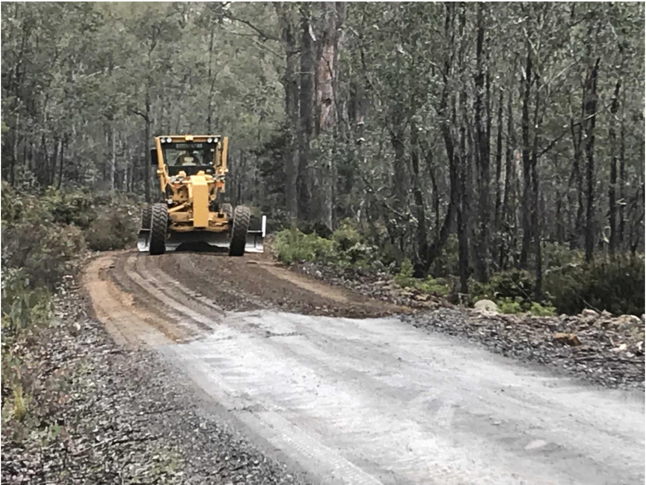
Grading material into Woods Lake Road
